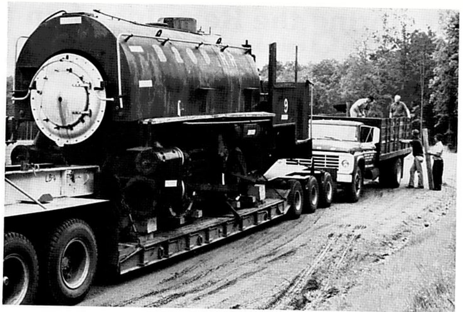
MAY, 1979: With tracks laid for loading, engine and wheels are placed on truck (above) at the locomotive's longtime resting place at Burnsville, N.C., in Yancey County. At right: Completing a route selected by the N.C. Department of Transportation to avoid low-hanging bridges, the dismantled locomotive arrives at Denton Airport.
